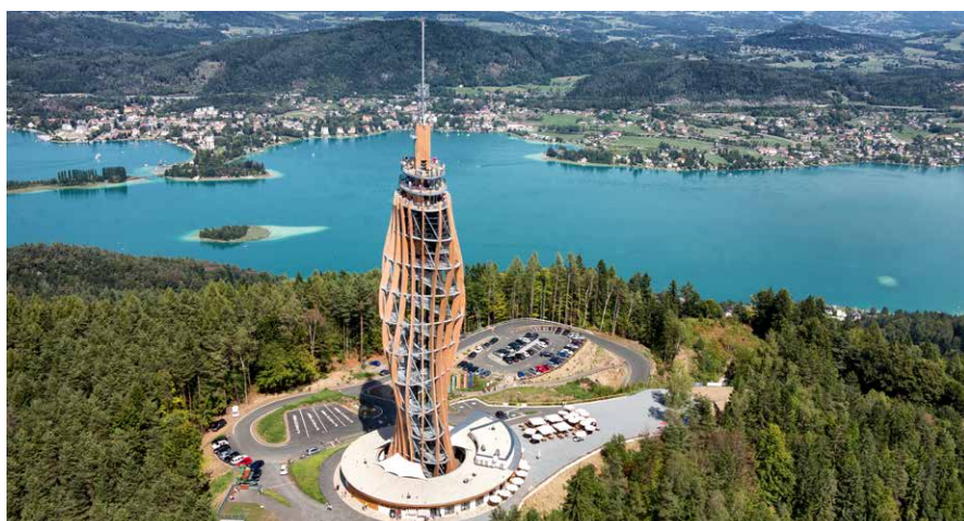
photos © Rubner Holzbau
