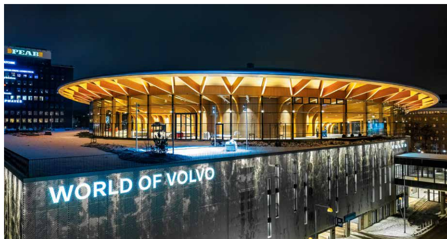
photos © WIEHAG Holding GmbH
