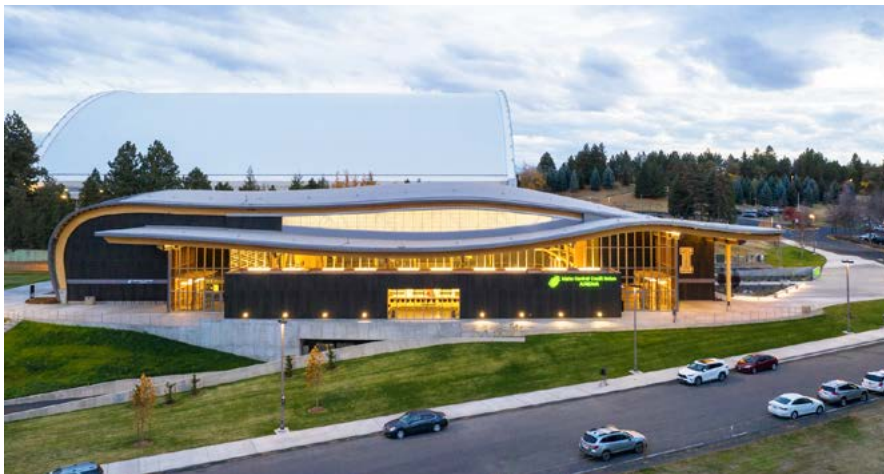
Photos © Structure Craft
